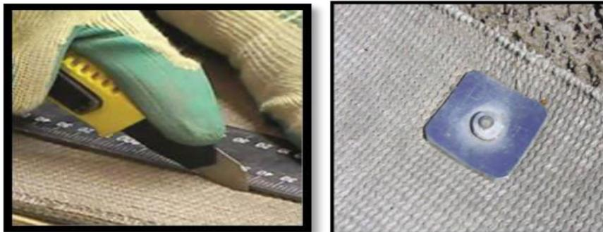
Fig3. Cutting and fastening of CC. (source- Milliken’s gallery)
