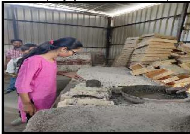
Fig.10.Placing of concrete in mould
