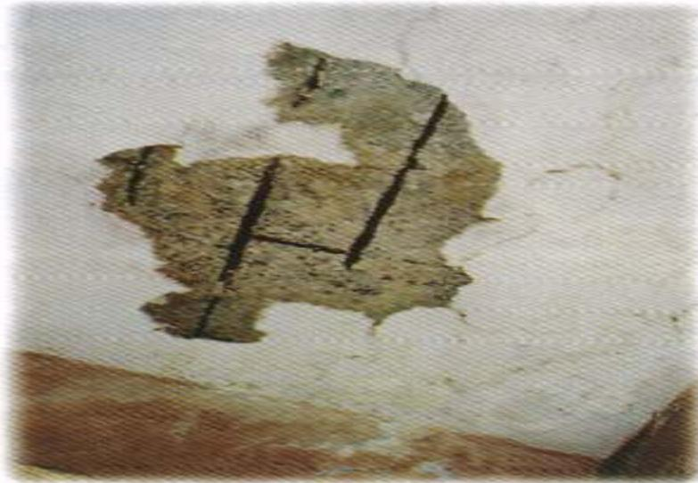
Fig.4. Corrosion of steel and spalling of concrete due to ingress of moisture
