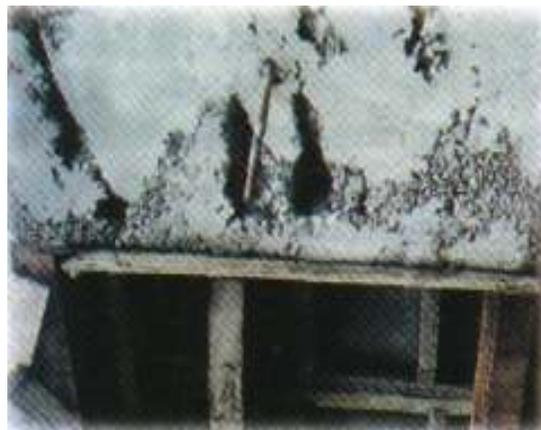
Fig. 6. Segregation of concrete causing honey comb
