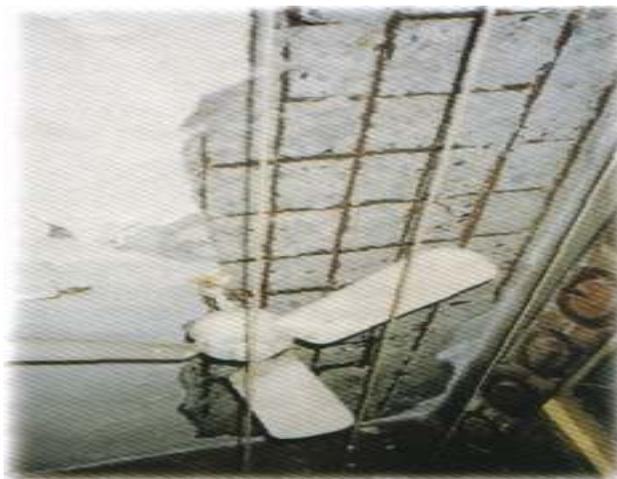
Fig.10. Spalled concrete due to corrosion of steel
