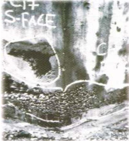
Fig. 2. Honeycombs at the foot of a RCC column
