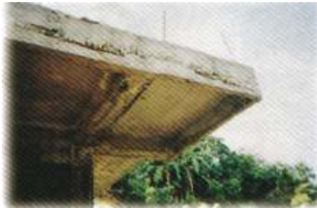
Fig. 7. Cantilever canopy showing honeycombing
