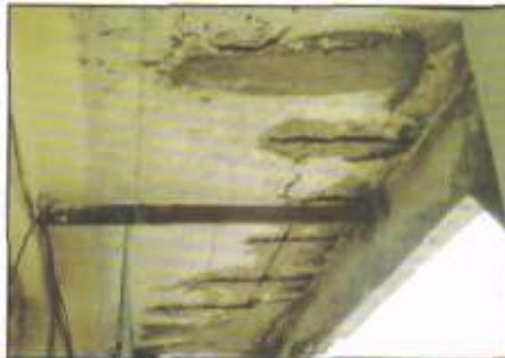
Fig. 5. Corrosion of steel in a canopy
