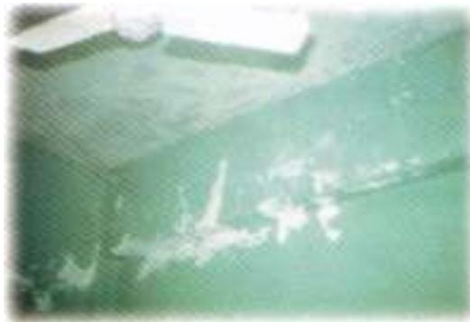
Fig.9. Leakage from roof slab
