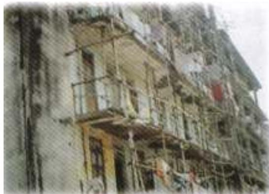
Fig.8. Badly deteriorated slender cantilever balcony slabs.
