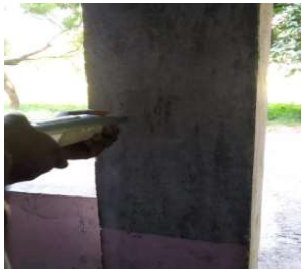
Fig.4.2.2 Testing on Column
