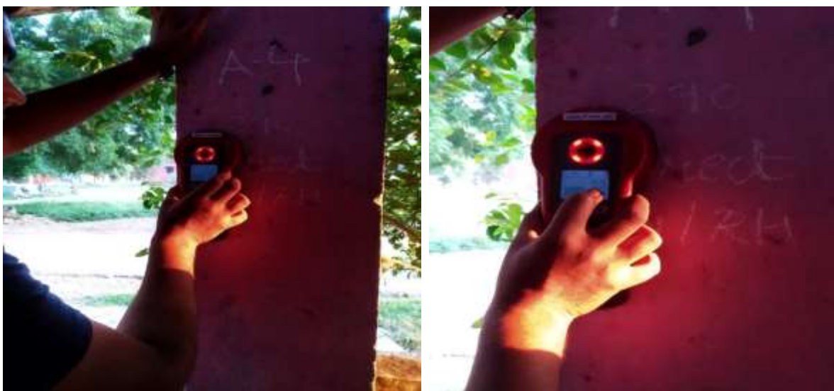
Fig. 4.6.1 Cover Meter Testing
