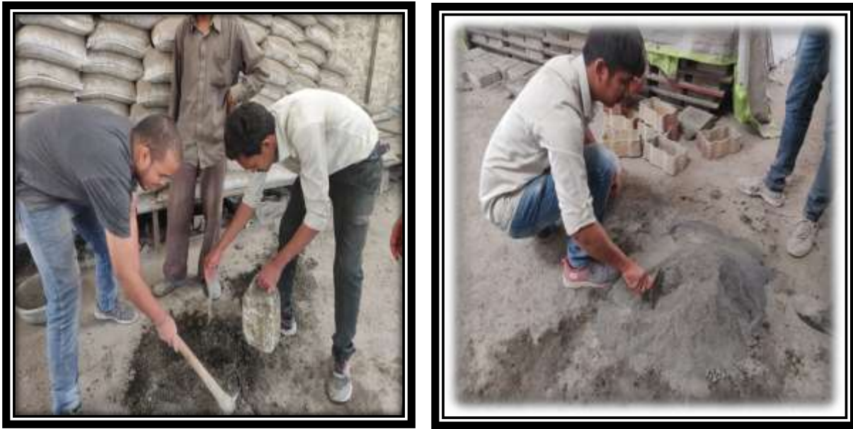
Fig. 6 Mixing of Materials
