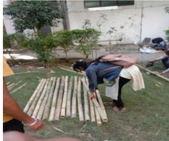
Fig 2- arrangment of bamboo for roof
