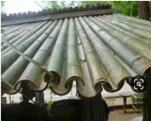
Fig 4- Sample of bamboo roof
