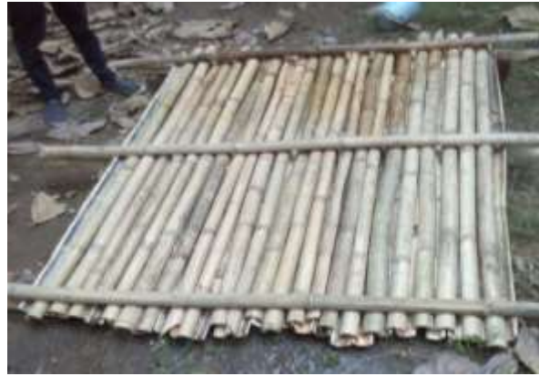
Fig 5- Construction of bamboo roof
