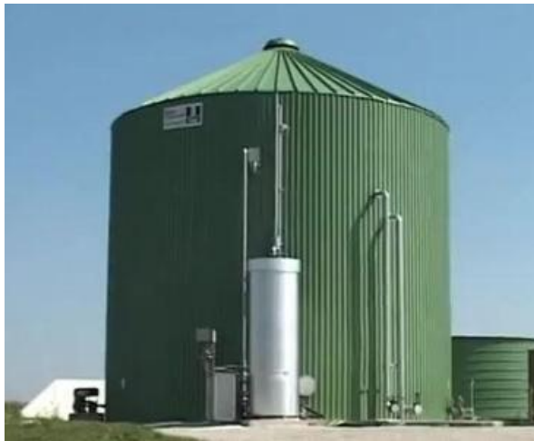
Fig.1. UASB reactor in Porur, Chennai
